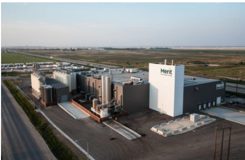
Figure 2: Merit Functional Food's new plant-based protein production complex in Winnipeg, Manitoba, Canada.
